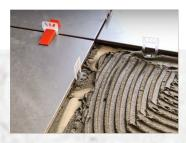
Set the adjacent tile firmly into the adhesive. Butt the tile against the clip giving the 1.0mm joint (if a larger joint is required spacers can be used, or set the required joint size).
