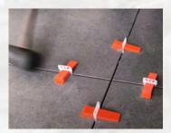
After the adhesive has set, you can remove the BATOFIX wedges and clips easily with a rubber mallet on the walls and by mallet or your foot on the floor.
