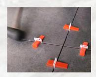
After the adhesive has set, you can remove the BATOFIX wedges and clips easily with a rubber mallet on the walls and by mallet or your foot on the floor.
