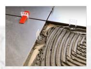
Set the adjacent tile firmly into the adhesive. Butt the tile against the clip giving the 1.0mm joint (if a larger joint is required spacers can be used, or set the required joint size).
