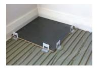
Spread your tile adhesive and lay the tile. Place the clips underneath the tile slightly back from the edge.
